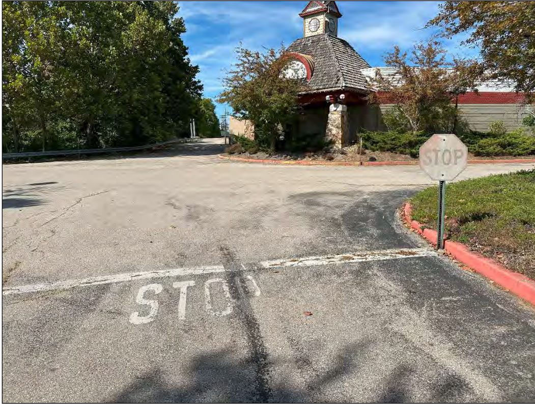
4540 Osage Beach Parkway – faded pavement markings and signage
