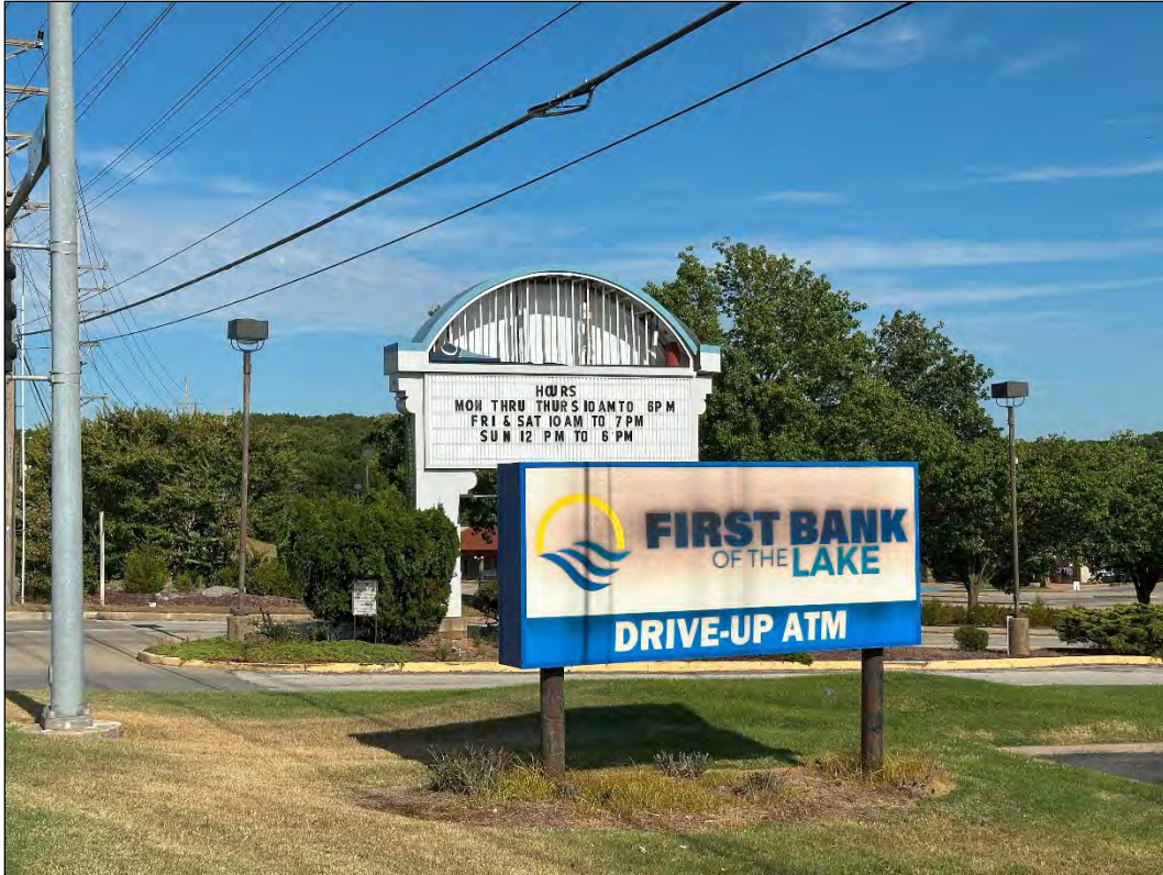
4540 Osage Beach Pkwy / First Office Centre – deterioration of signage
