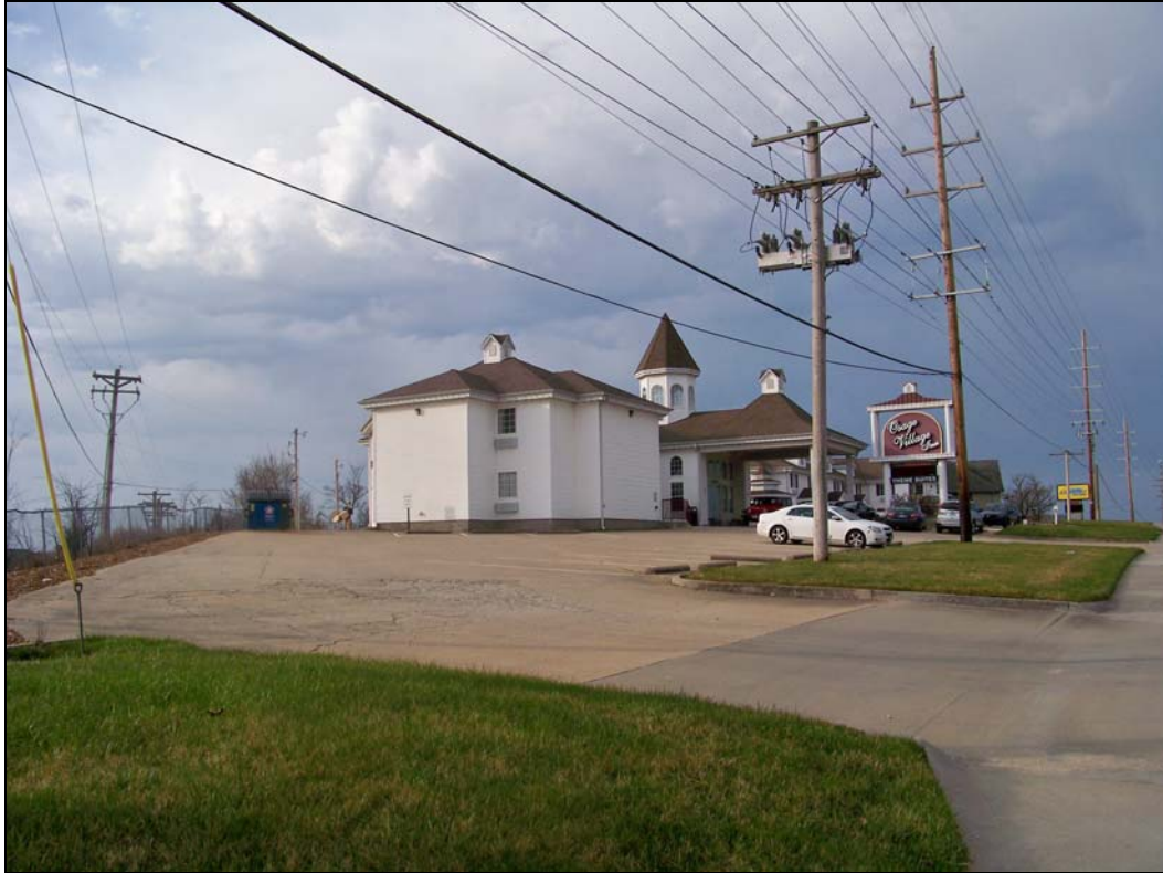
4540 Osage Beach Pkwy – looking west – deterioration of parking lot pavement
