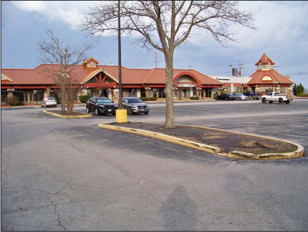
4540 Osage Beach Pkwy – looking west – neglected landscaping
