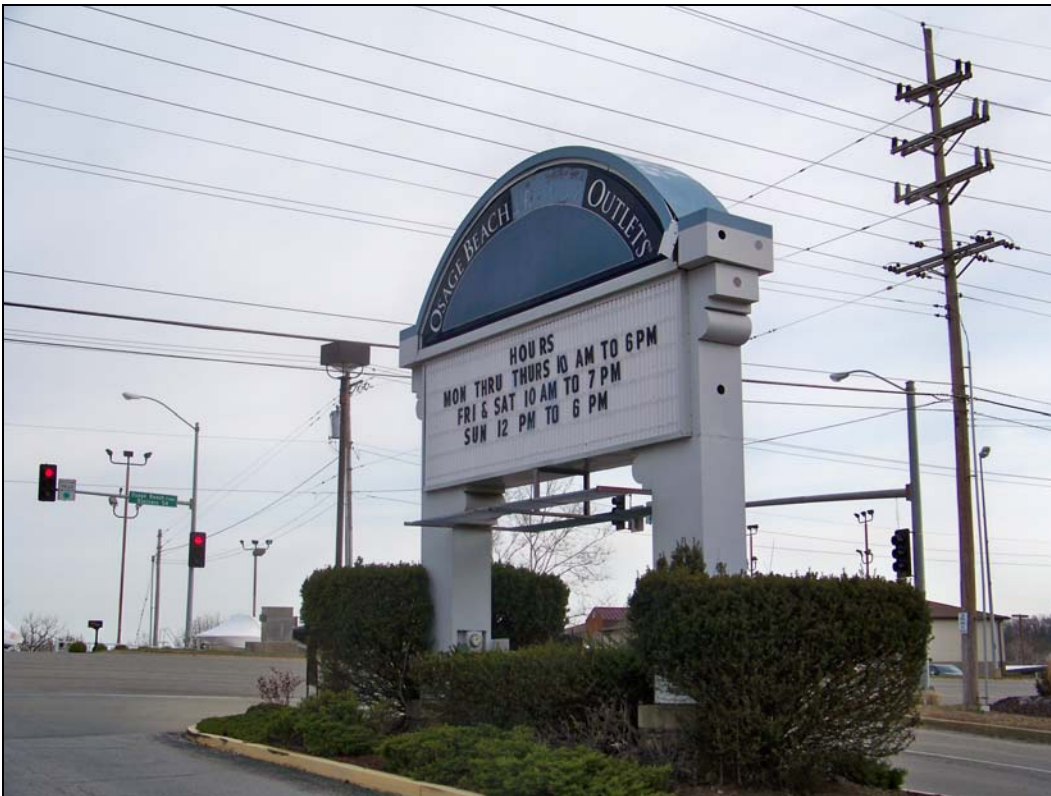
4540 Osage Beach Pkwy – looking north – deterioration of signage
