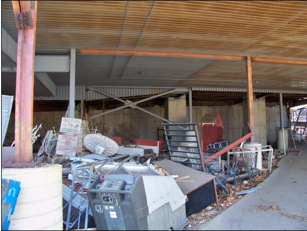
4540 Osage Beach Pkwy – looking west – trash/debris
