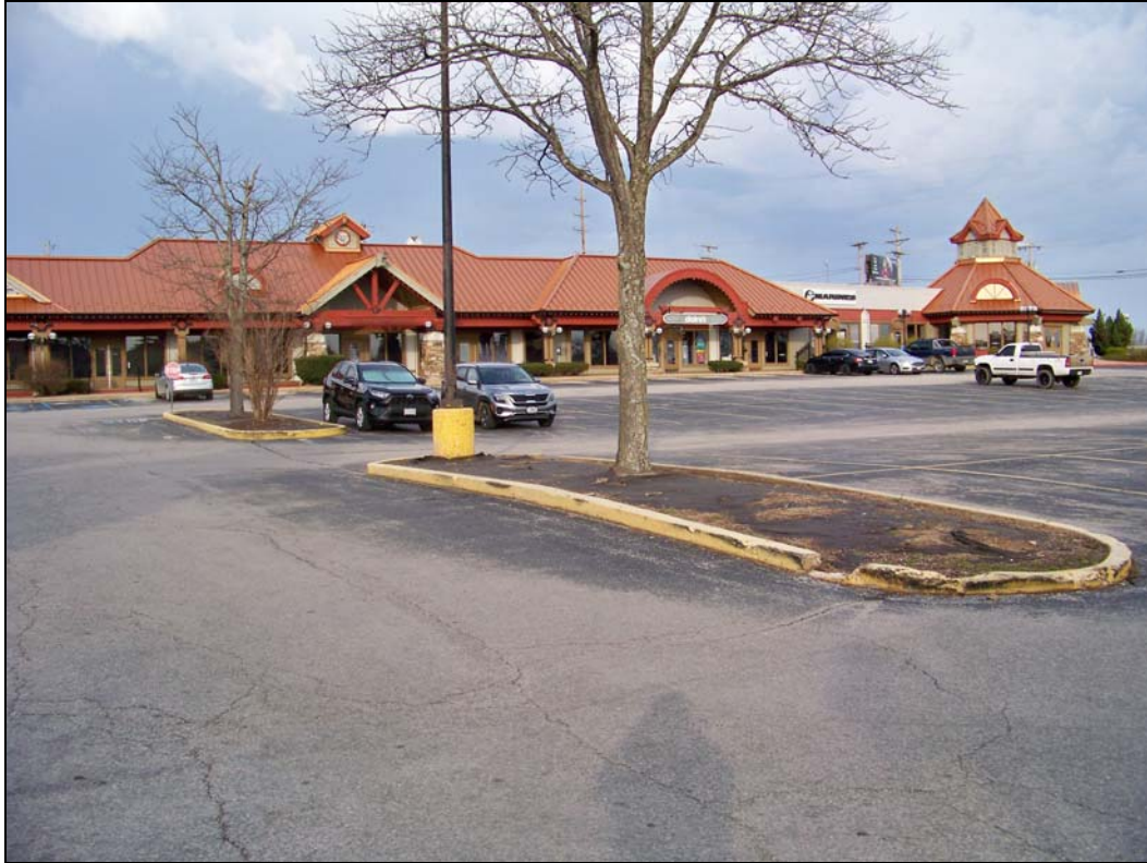
4540 Osage Beach Pkwy – looking west – neglected landscaping
