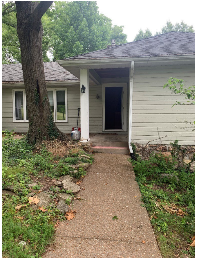
Above: Open and unsecured vacant home.
