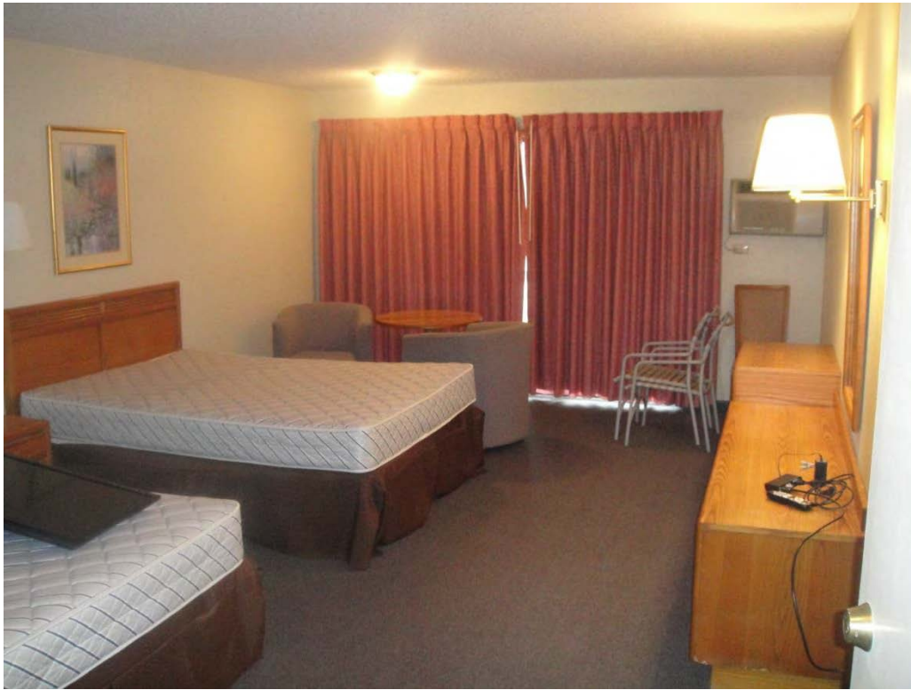
Typical room furnishings throughout hotel and villa facilities. All finishes not in compliance with current Best Western design standards.
