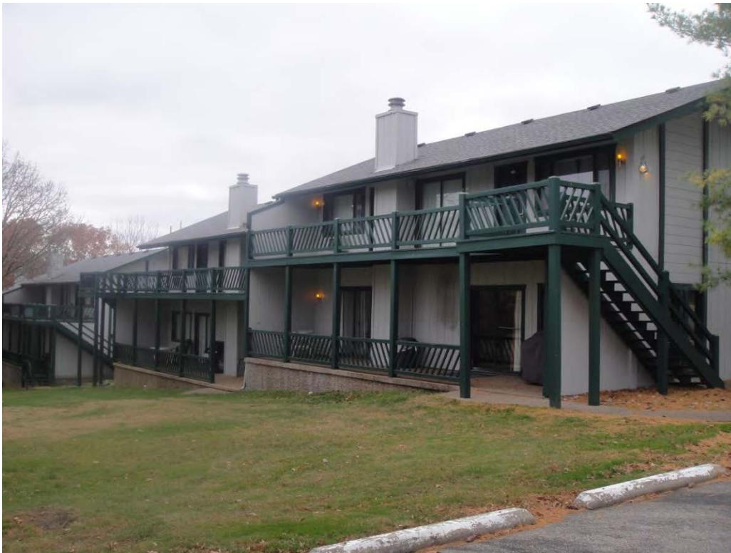
East façade of the four villa buildings. Note exterior stair access.
