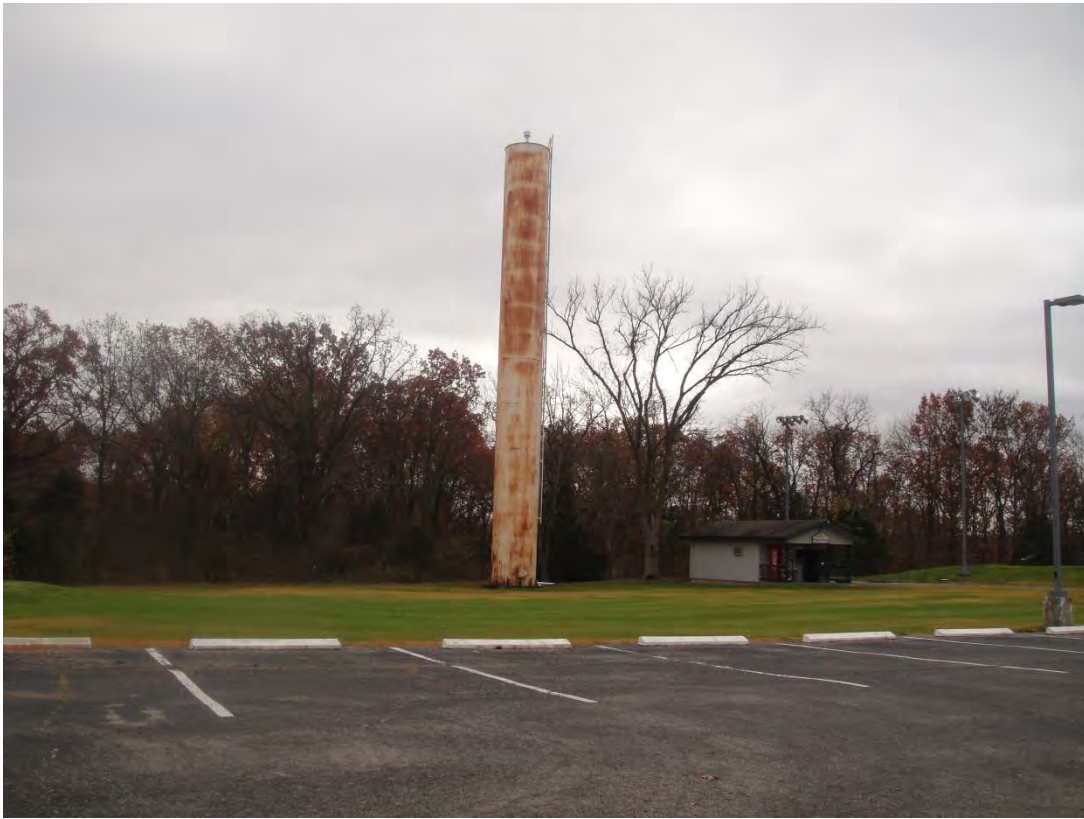
View of 30,000 gallon Standpipe water tower.
